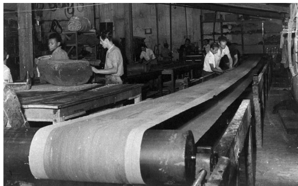
Figure 6. Early belt conveyor [13]
